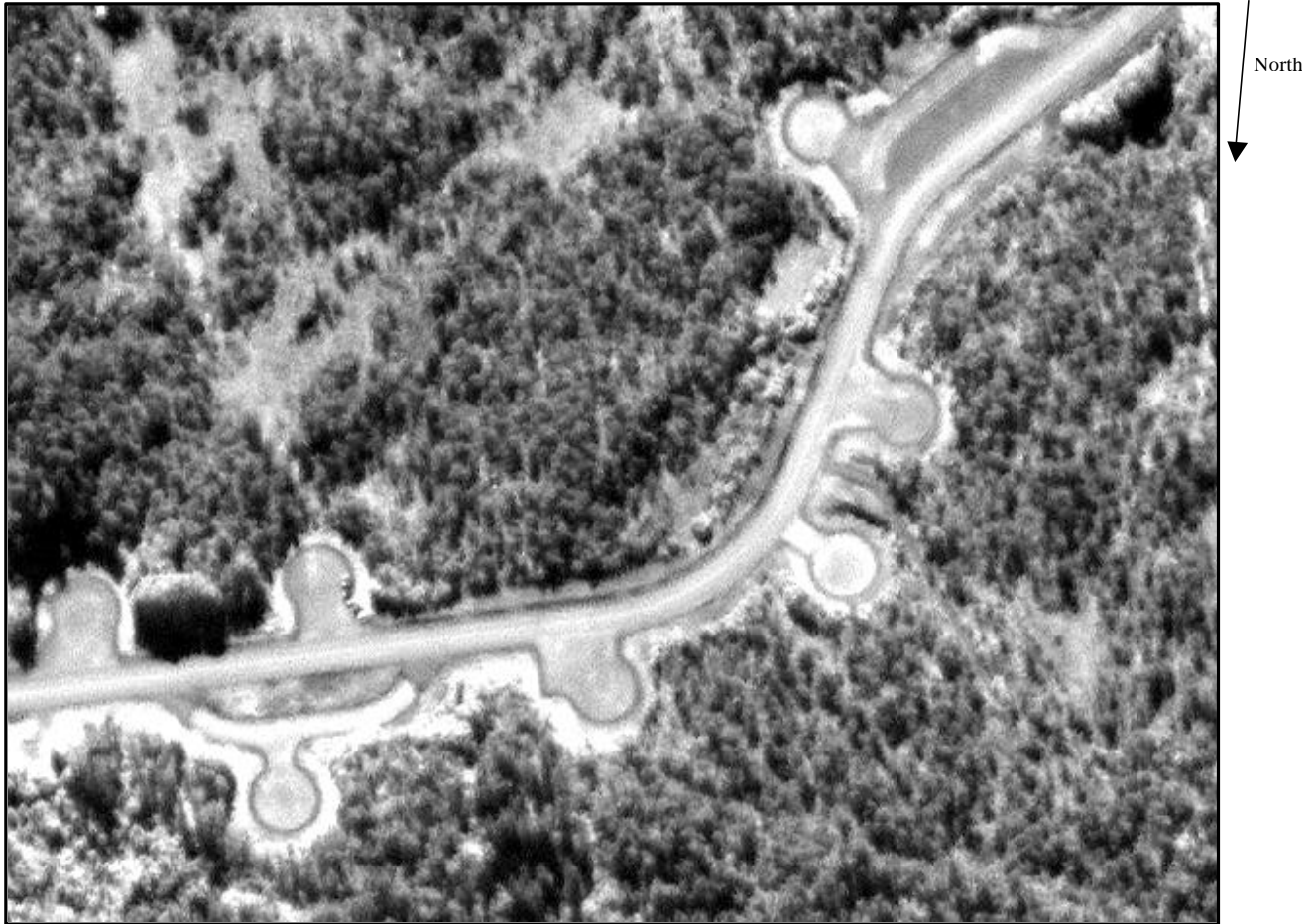
Figure 5.33 Road/taxiway detection at Tjukkehovden. IKONOS.
