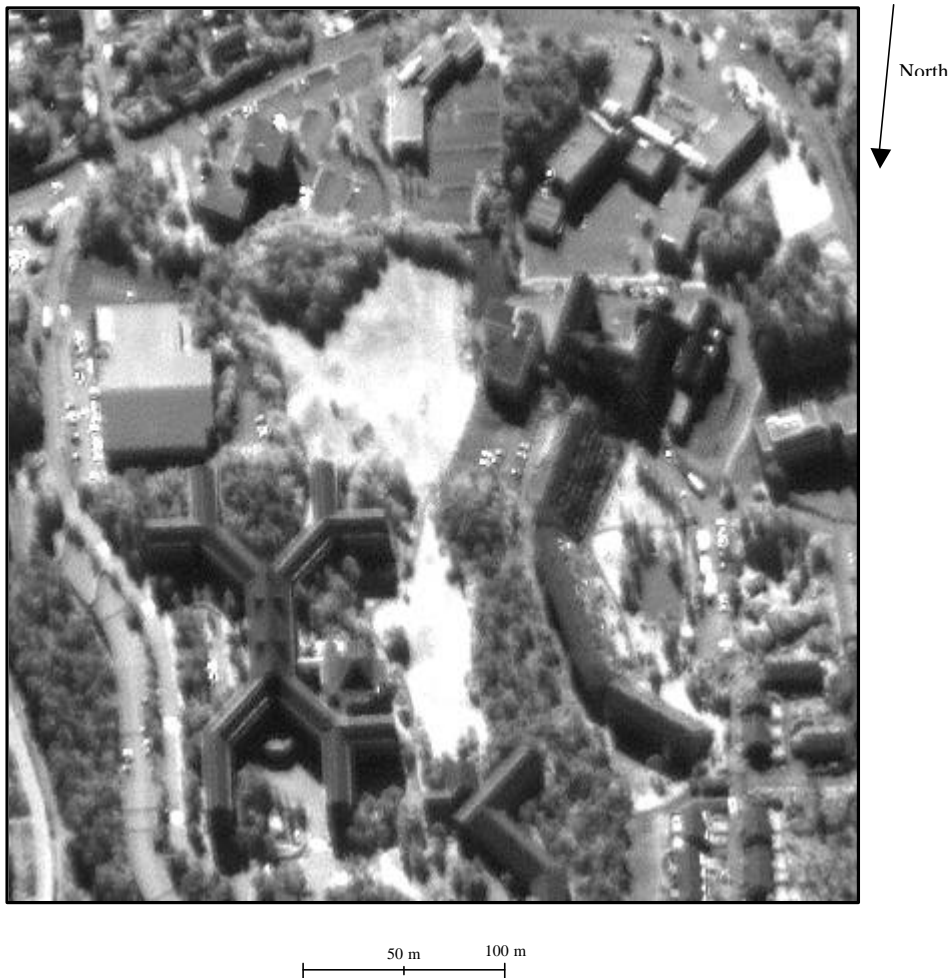
Figure 5.25 Complex shaped buildings at Sandsli Kjeldsnet. IKONOS
