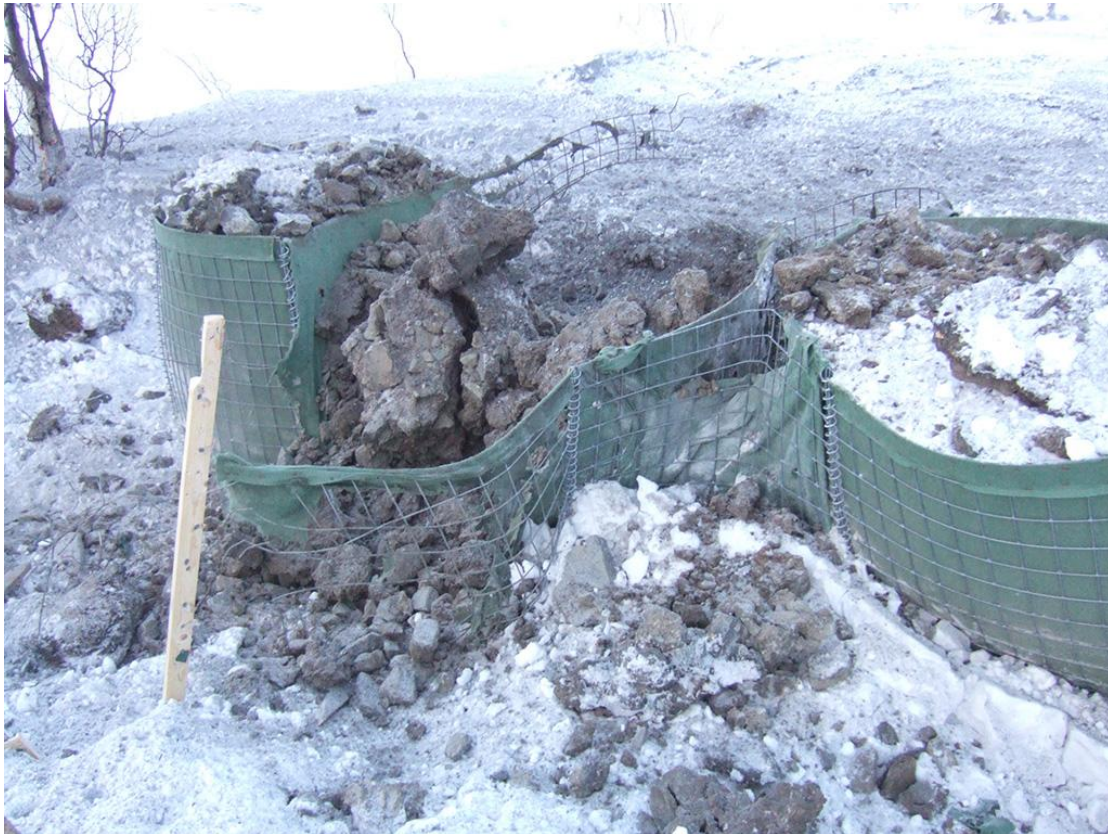
Figure 2.13 Back side of wall after test 1.4
