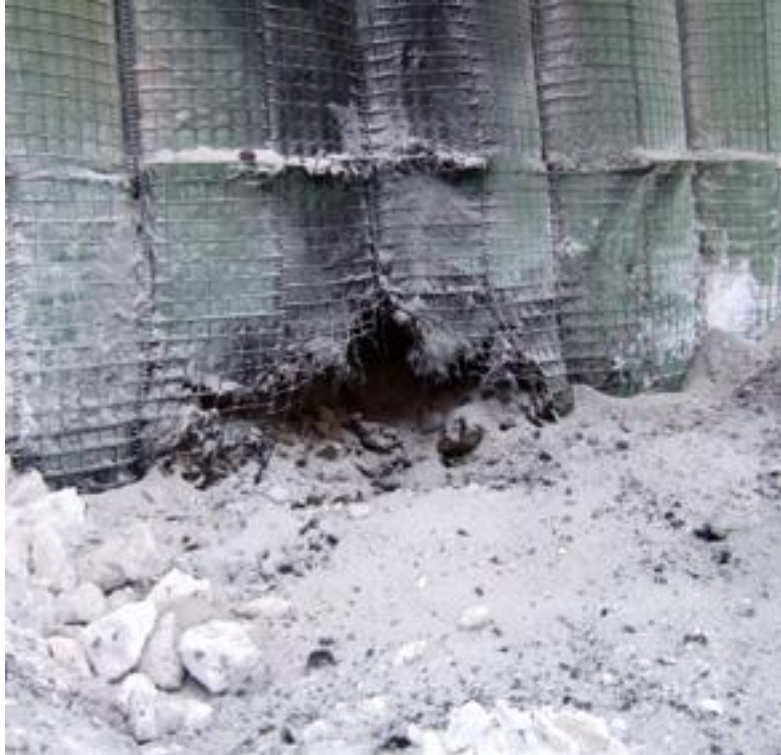
Figure 2.26 Crater in the wall after test 2.4
