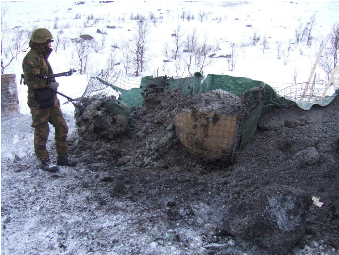
Figure 2.10 Front side of wall after test 1.3
