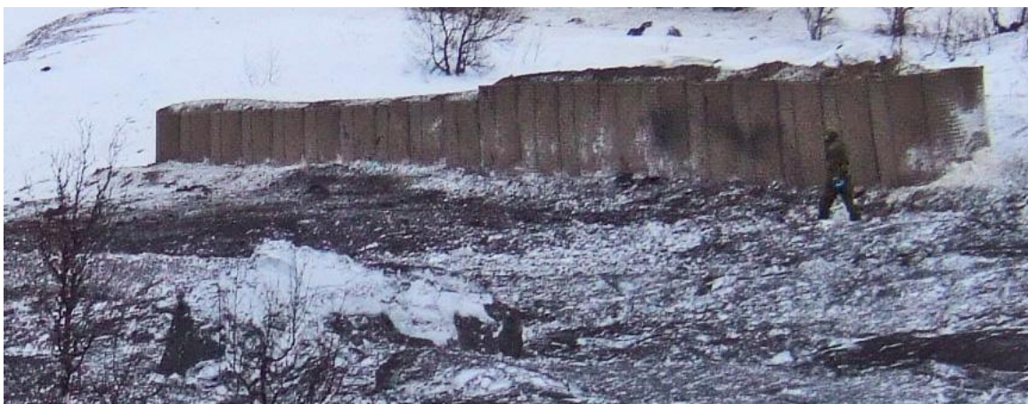
Figure 2.28 MIL 10 walls after test 3
