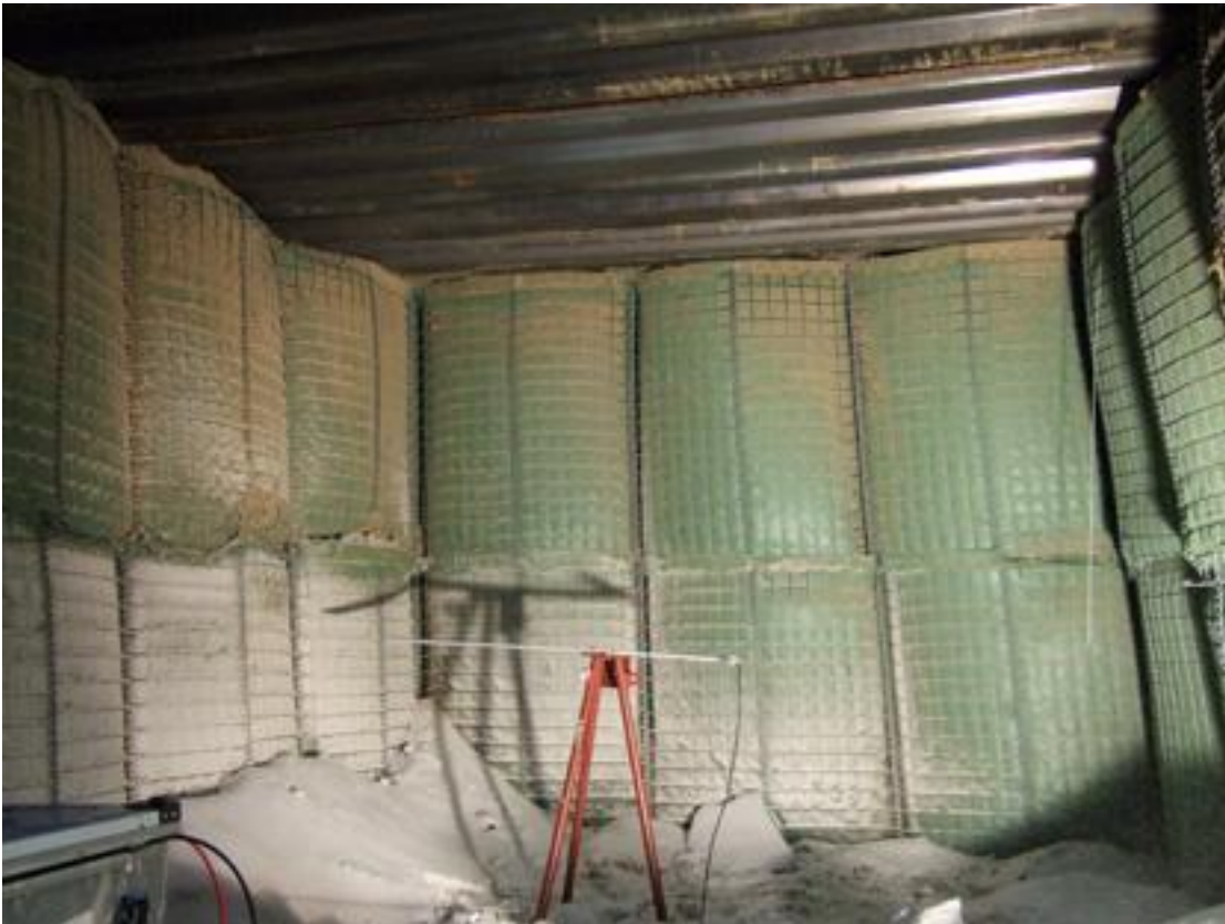
Figure 2.20 Inside of UTOPS shelter
