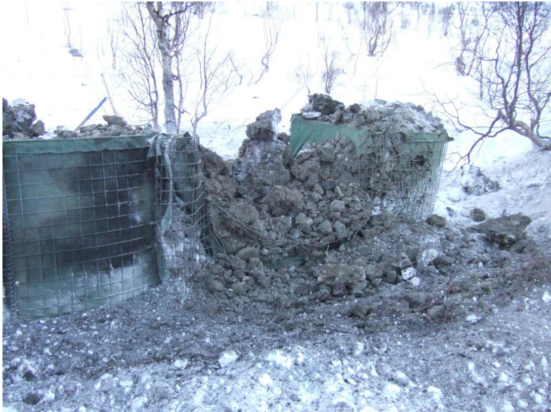
Figure 2.12 Front side of wall after test 1.4
