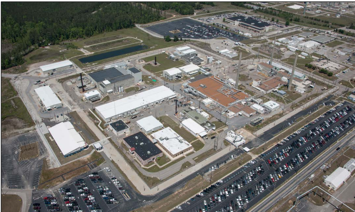
Figure 3.1 Savannah River tritium facilities at the Savannah River Site in South Carolina, USA. (Picture from Ref. (4).)
