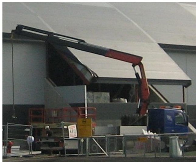
Fig. 5. Sports hall north of Lillestrøm city centre. Top: Two of the TSX images acquired with 37° and 47° incidence angles. Note the arches that are shown up with bright backscatter in the SAR images. Copyright SAR data: TSX 2008, DLR. Middle and Bottom: Photos of the sports hall with the sandwich roof being mounted (D. J. Weydahl, FFI).
